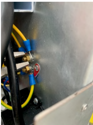
Ensure all terminals and earth connections are tight
